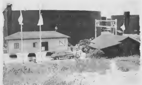
The old Electrical Training Building starts out the gate to the Anglican Church in San Nicolas, to become a parish social center and meeting place for British Scouts and Girl Guides. This is one of several buildings that Lago has given to Church or Scout groups on the island.
